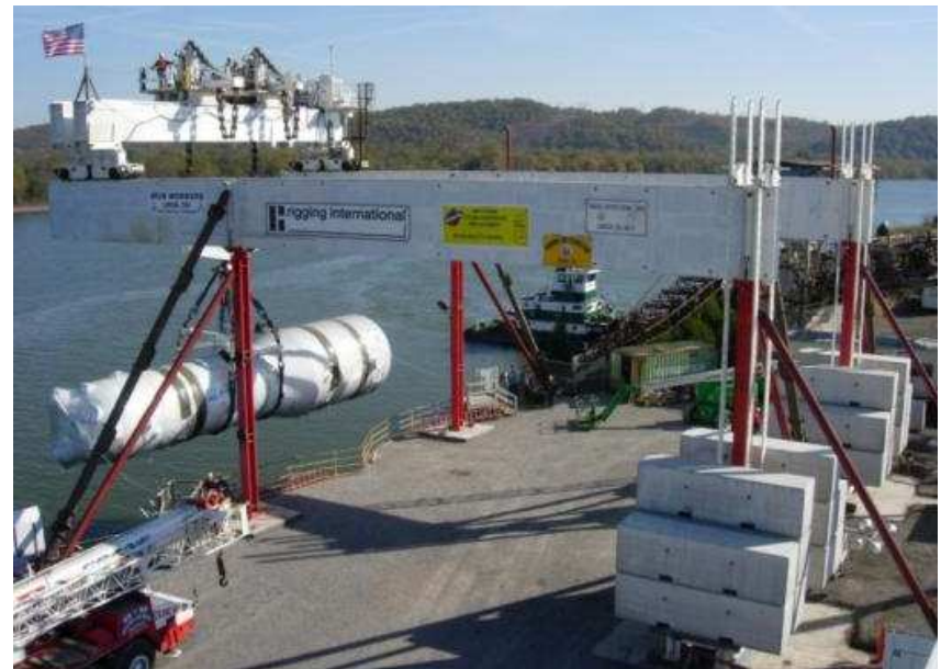
Cantilevered steam generator offloading system, Watts Bar
